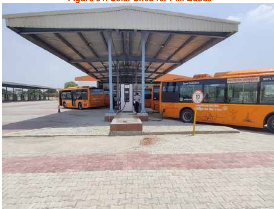
Figure 34: Solar Shed for PMI Buses
