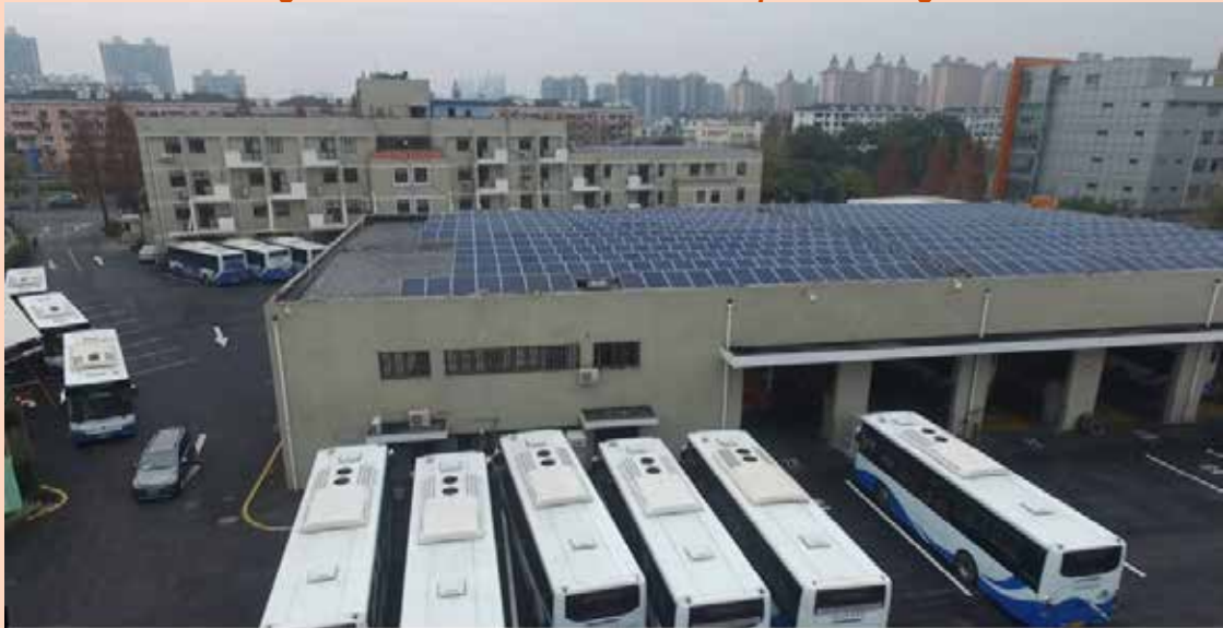
Figure 35: Solar PV Powered Bus Depot in Shanghai
