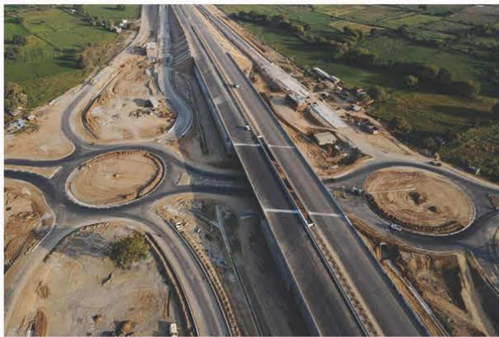
A section of Bundelkhand Expressway in Uttar Pradesh (UPEIDA)
