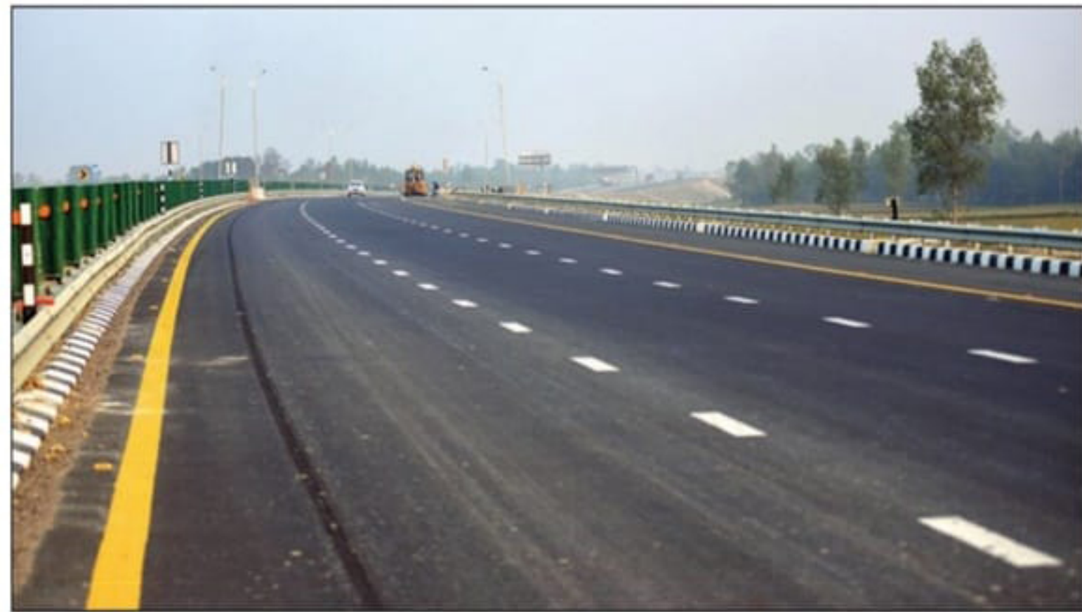
ROAD TO DEVELOPMENT: New expressways will expedite growth in state
