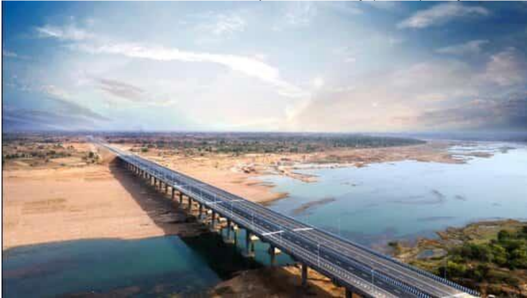
A view of the Bundelkhand Expressway. (Sourced)
