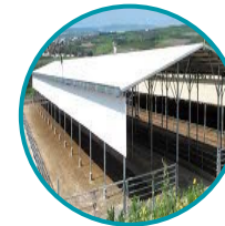
Development of storage infrastructure
