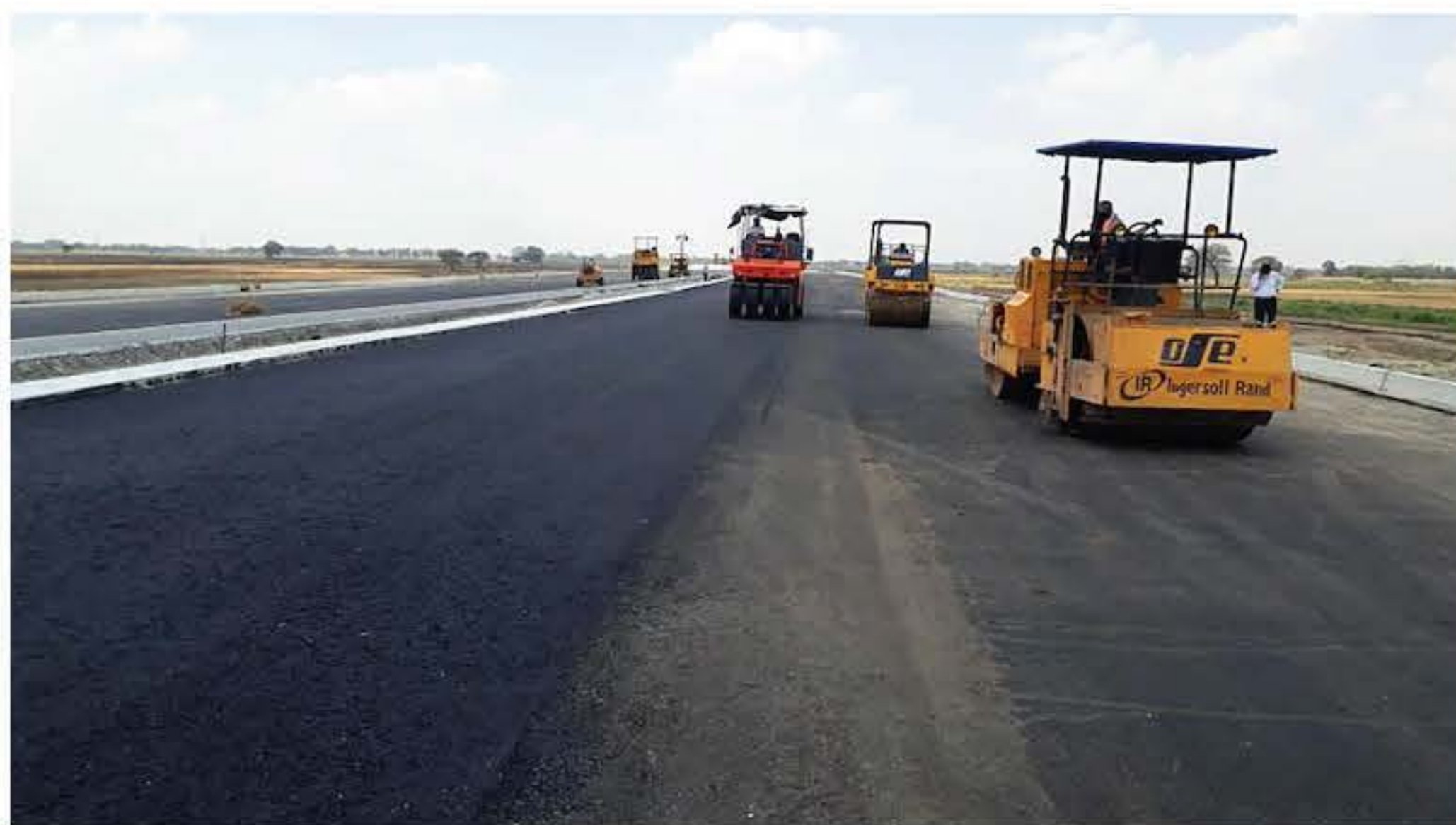
Construction work on the Purvanchal expressway, in May (ANI)
