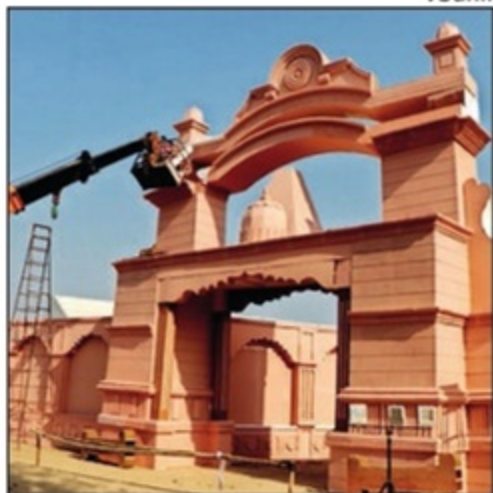
Ayodhya tent city work in full swing at Vrindavan Yojana
