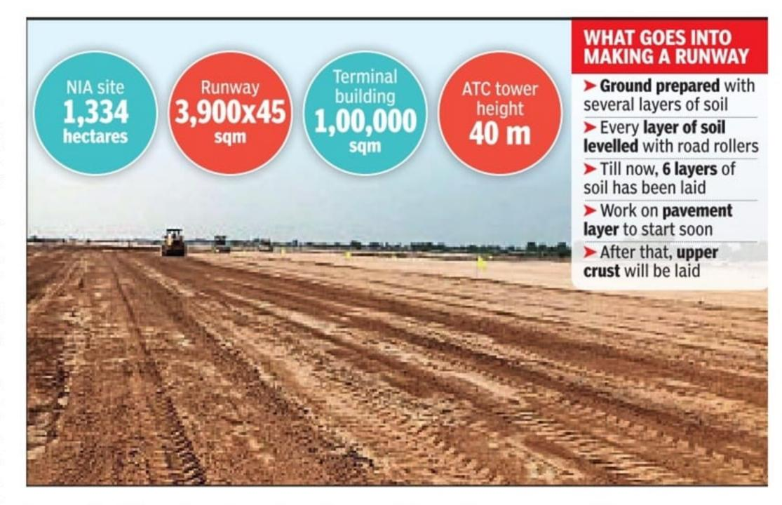
layers of soil have been levelled with road rollers. Work on the 'pavement layer' will start next, followed by the upper crust. Once the lighting is done, the runway would be ready.
