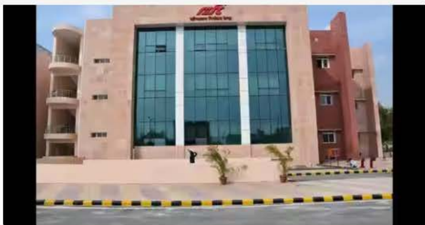
EDFC control room set up in Prayagraj (HT Photo)
