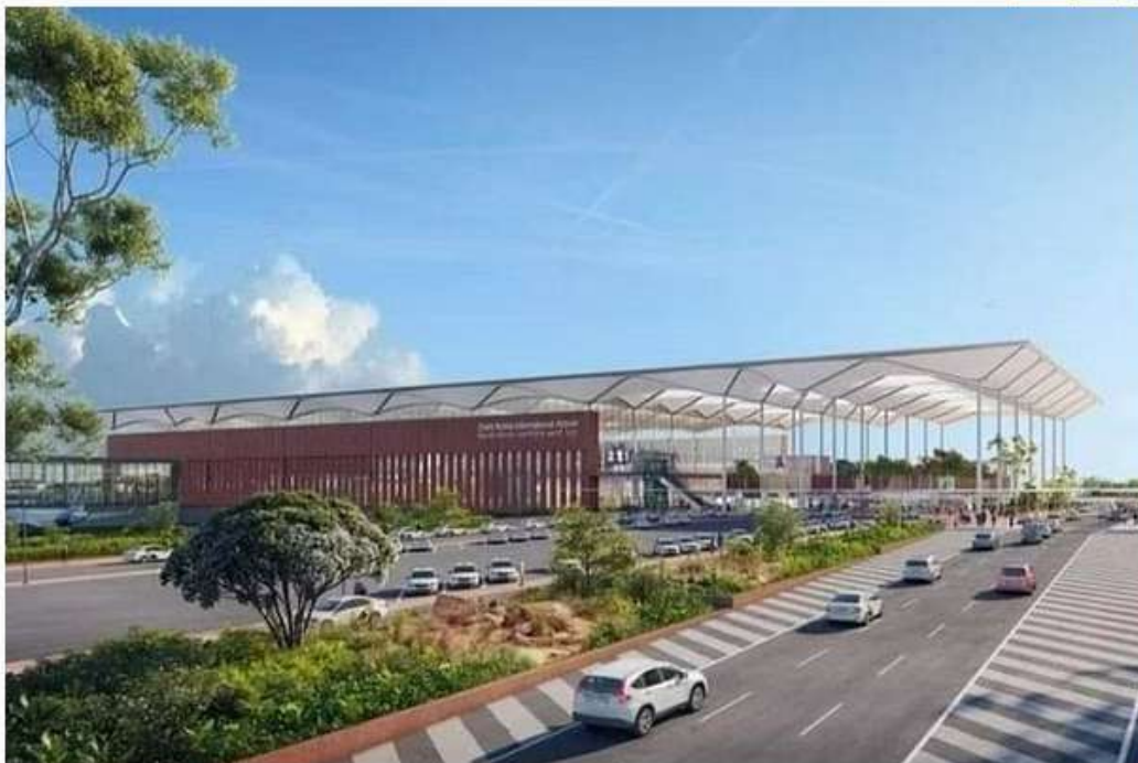
An illustration of the proposed Noida International Airport at Jewar in Uttar Pradesh.
