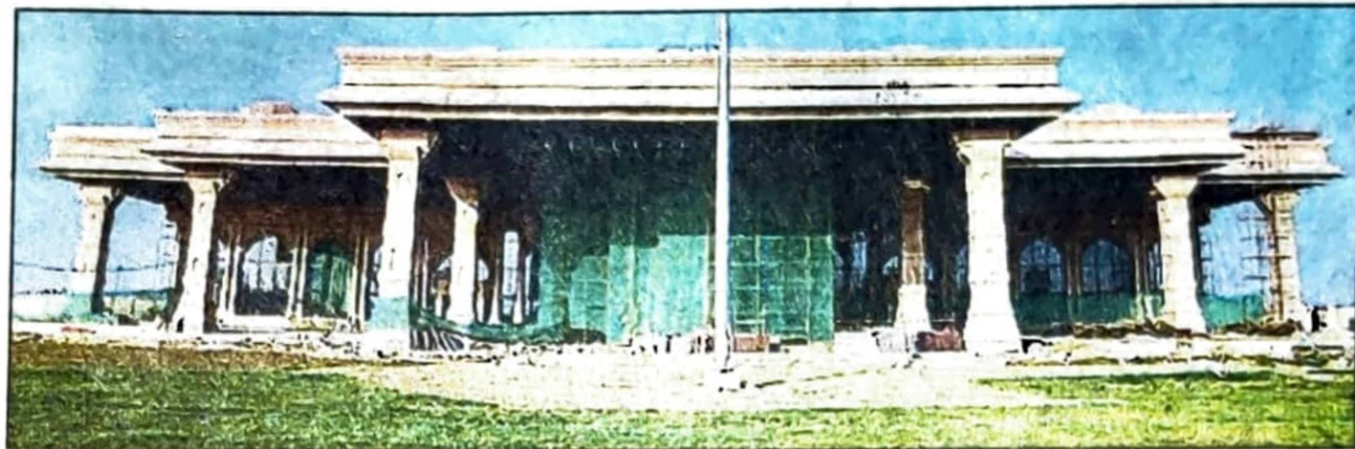
International airport under construction in Ayodhya
