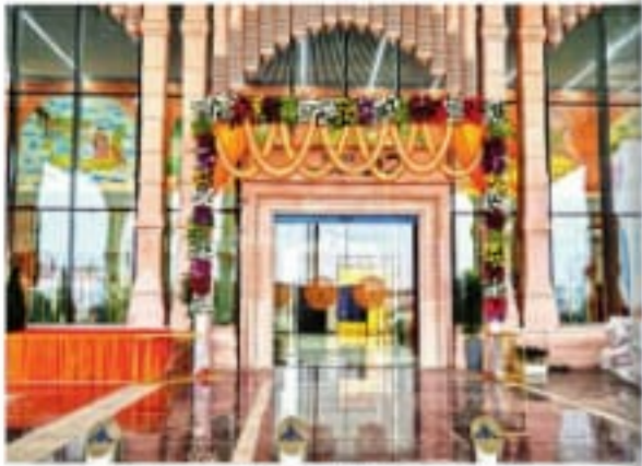
Maharishi Valmiki International Airport, Ayodhya
