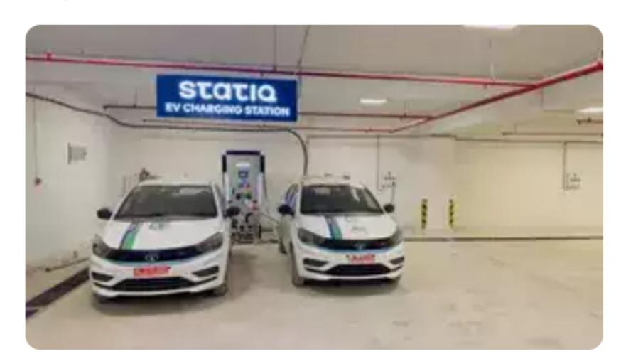
The charging station is equipped with one 60 kW DC charger (dual gun) and four 9.9 kW AC chargers, each featuring three sockets of 3.3 kW.
