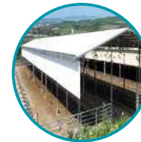
Development of storage infrastructure
