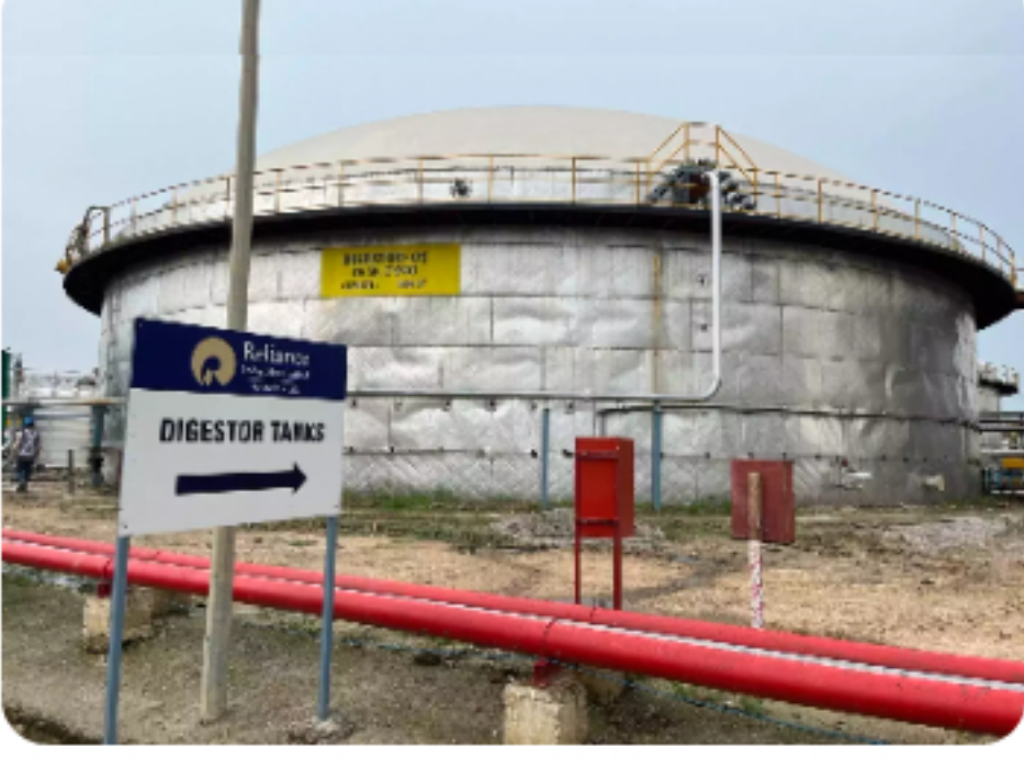
Each CBG plant is designed to handle between 250 and 500 tonnes of feedstock daily, producing 10 to 20 tonnes of CBG.
