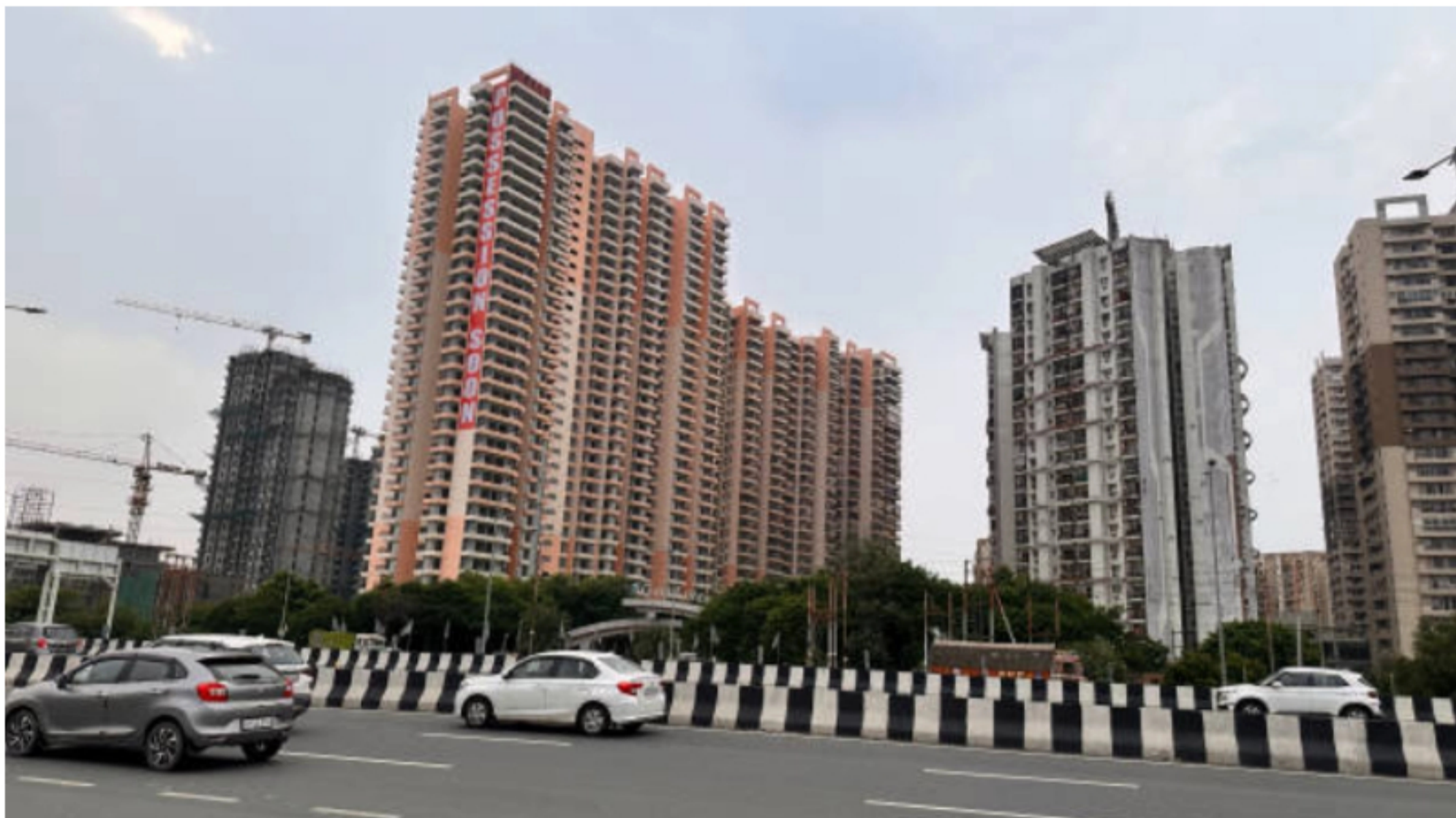
Roads, Parks, and Streetlights! Ghaziabad Prepares for Major Infra Revamp in 10 Industrial Areas (Representative Image)
