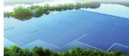
400 MW Metalia dam & reservoir floating solar project; 37 MW Jamini dam & reservoir floating solar project, Lalitpur; 27 MW Arjun Sagar floating solar project, Mahoba
