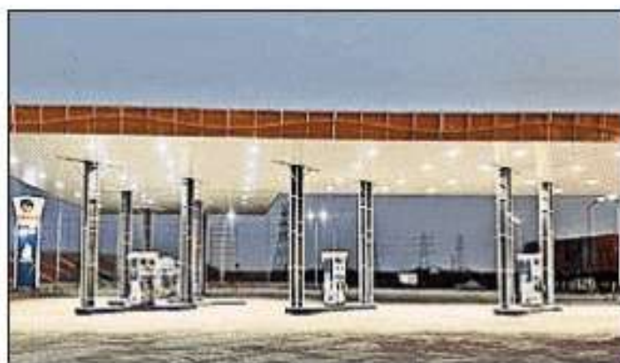
Petrol pumps ready for operations at Ganga E-way
