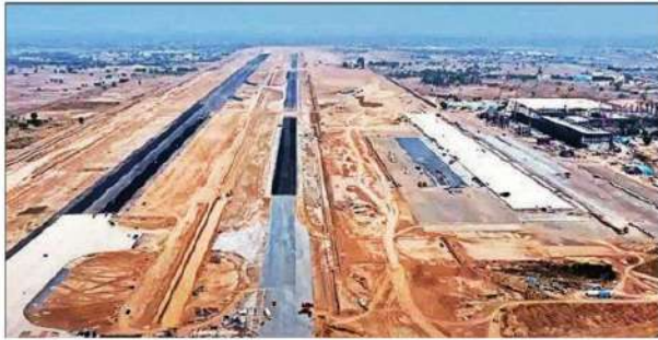
A review of new expressways was held on Thursday
