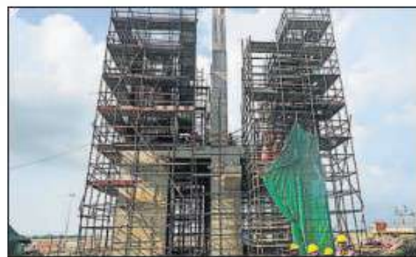
Ongoing facade work on the terminal building.
