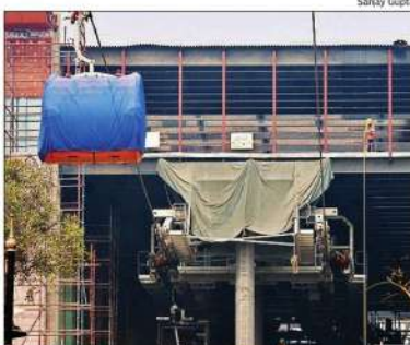
Alignment test of ropeway being conducted in Varanasi on Thursday
